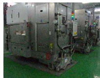
切割车间 Cutting Workshop
